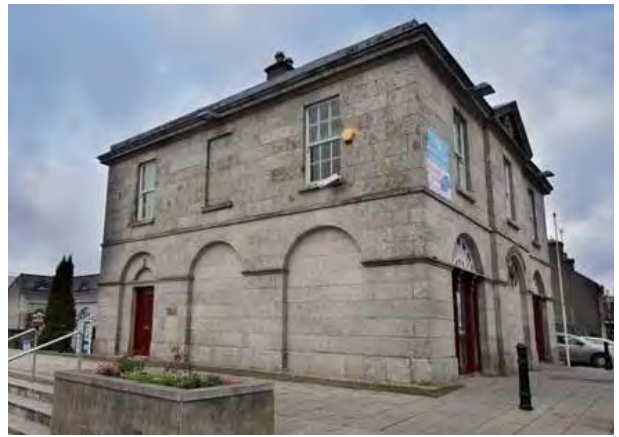
Figure 40 The Credit Union building and Monument provide an architectural flair to the Square
