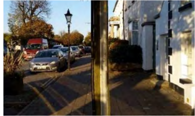
Figure 38 Example of poorly placed service poles
